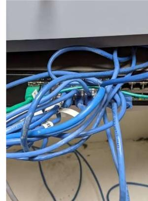
We recommend replacing the existing cable runs entirely, new cables to be run inside walls / above ceilings where possible and installed in raceways if necessary. All cables should be brought back to a single central point. All cables should be labeled clearly at both ends for ease of identification and, at the server end, cables should terminate in a patch panel.
