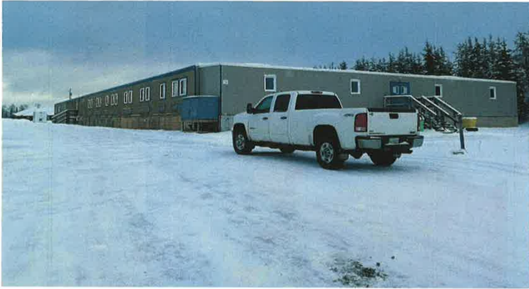
Temporary Bunkhouse located at 714 Rue de l’Eglise – Owned by Alamos Gold Inc.
