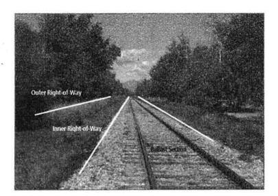
Vegetation in the right of way section needs to be controlled to protect sight lines for train crews to see signal systems and at road crossings, prevent trees from fouling the track during storms, reduce fuel loading to prevent fires, minimize wildlife mortality, ensure
